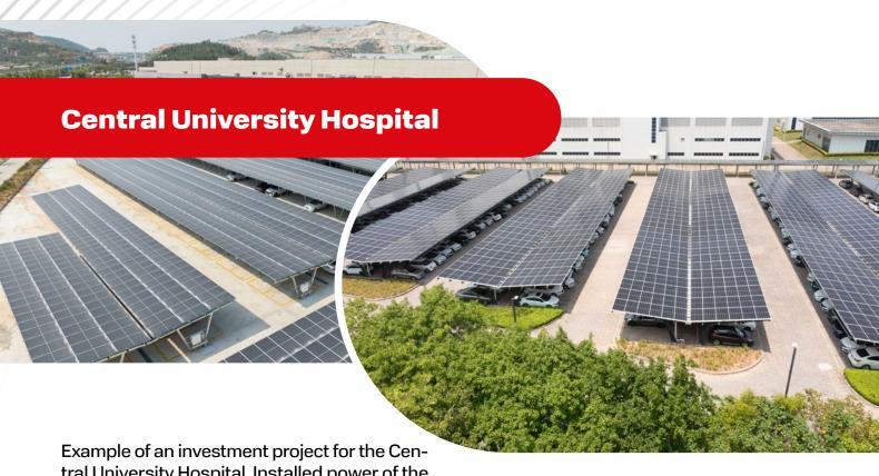
Example of an investment project for the Central University Hospital. Installed power of the photovoltaic system of 2.45MW over an area of 13,000 m² makes it possible to generate electricity without restricting the parking area. The use of multiplied carports at public facilities brings tangible benefits for both investors and users.
